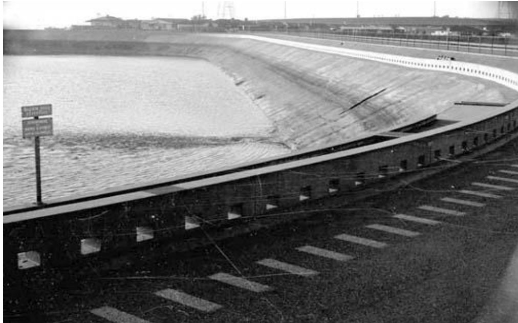
Baldwin Hills Dam - Dark spot in upper right hand quadrant shows the beginning of the break in the dam.
